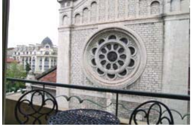
View from lounge balcony
